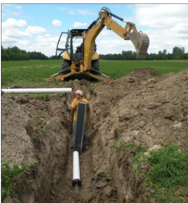
Figure 2: Installation of a water control structure.
